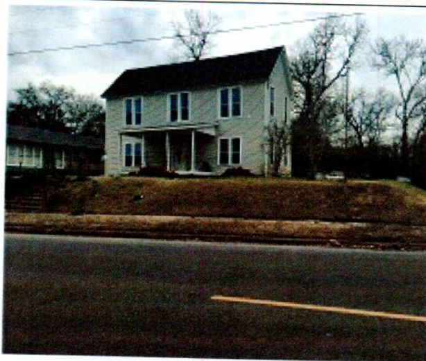
Single family residential and commercial to the north
