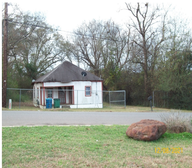
Single family residence to the north
