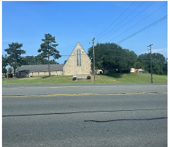
Church to the south
