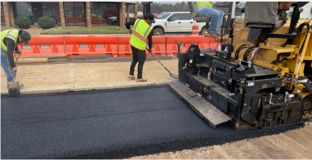
Infrastructure improvements on State Highway 80
