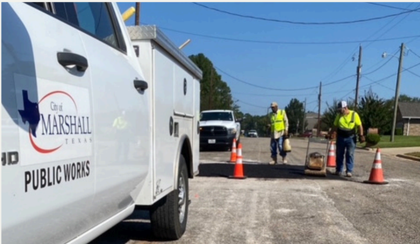
Public Works crew members maintaining streets
