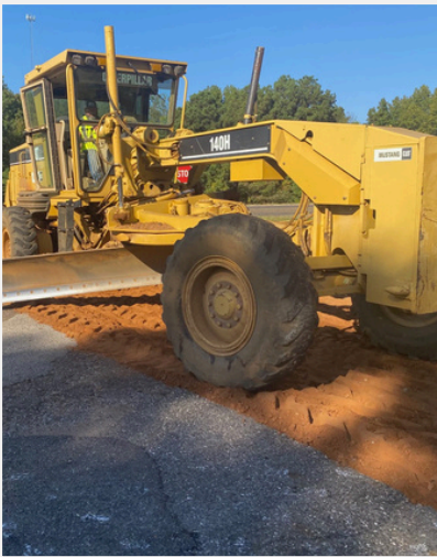
Roadway construction on Scotts Quarter Road and Hudson Street
