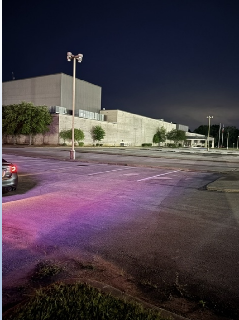
Convention Center Parking Lot Lighting _ 2026
