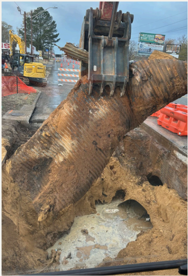
Replacing aging pipelines
