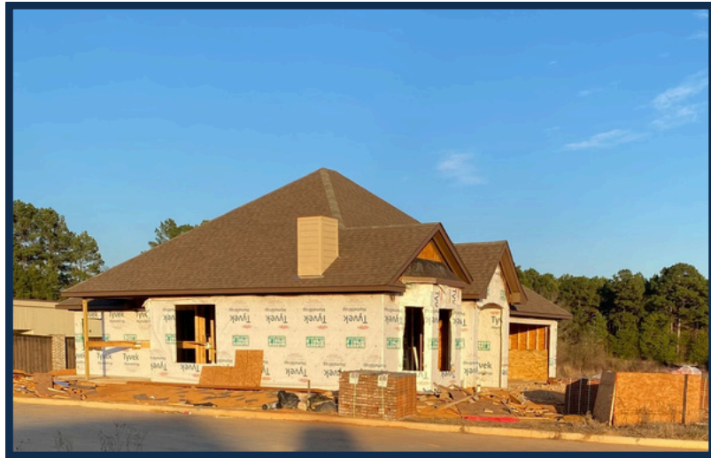
New home construction in 2025 near Airport Park.
