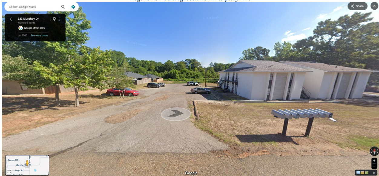
Figure 3: Looking North on Murphey Dr.
