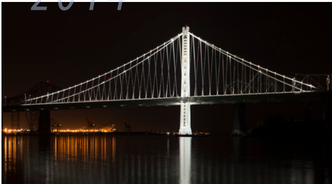
Our Team designs a state-of-the-art LED system for installation at the East Span of the San Francisco-Oakland Bay Bridge , improving driver safety and energy efficiency.
