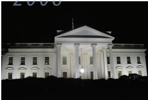
Our Team completes the first LED installation at the White House, lighting the external façade and cutting energy consumption by 87%.
