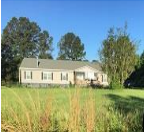
Single family residential to the East
