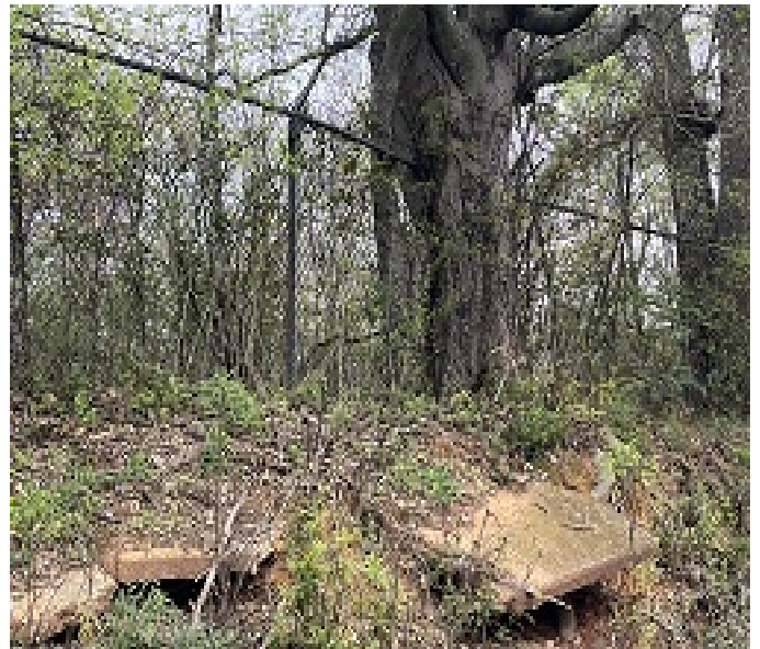
Vacant Commercial to the west
